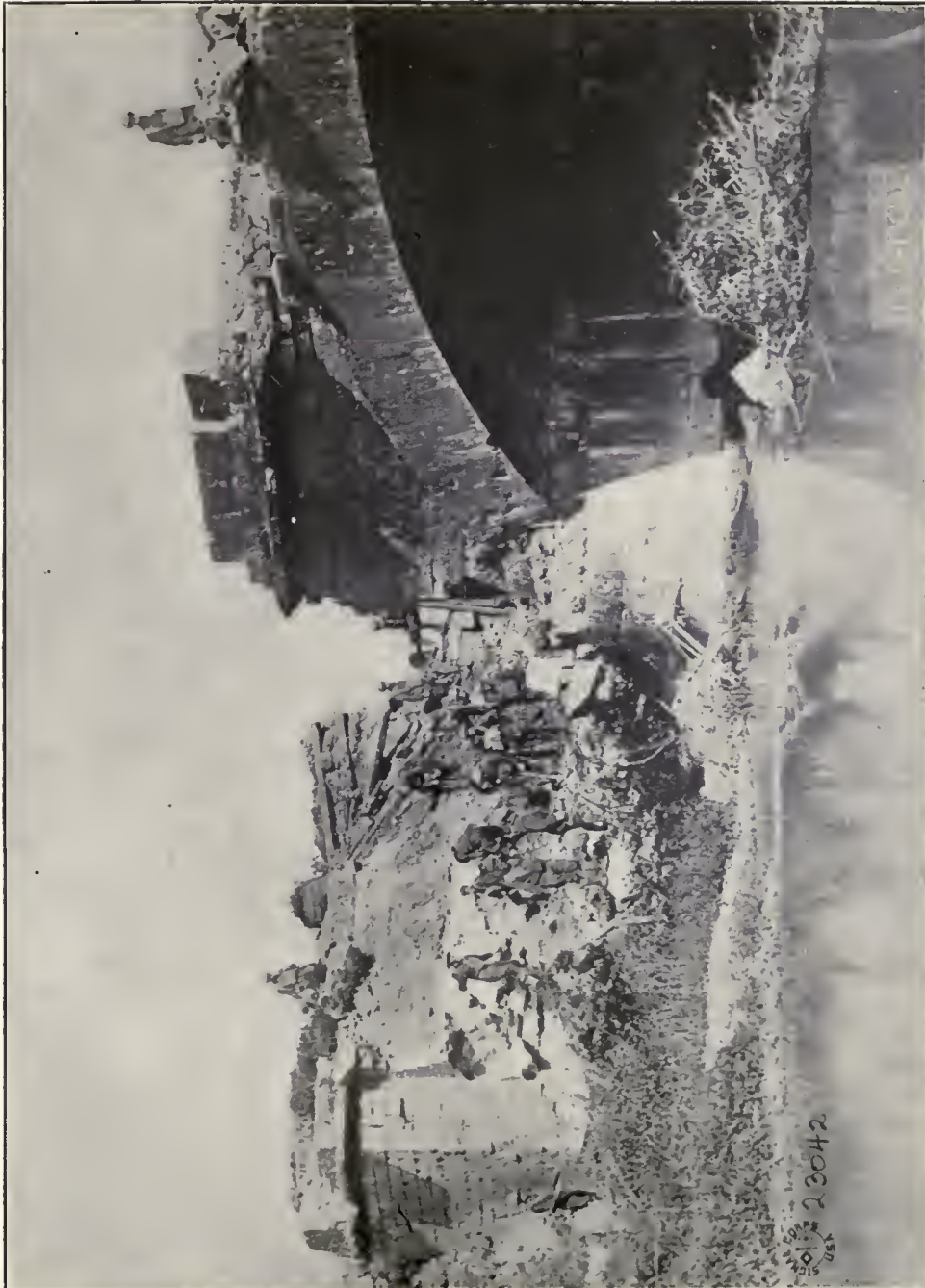
American engineers at work replacing a bridge across the Aire which had been dynamited by the Germans after retreating before the Franco-American assault.
